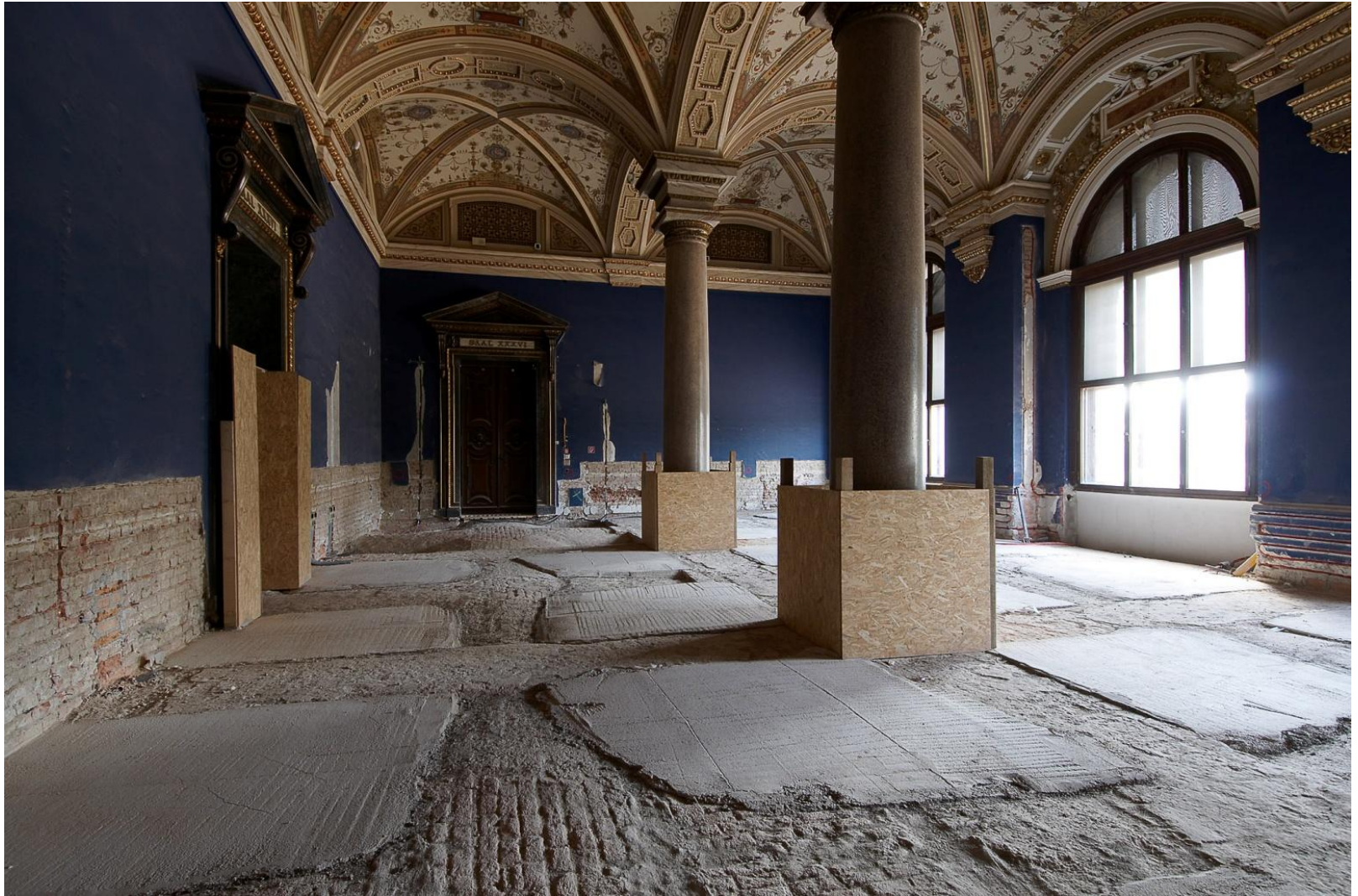
Room 36, during Renovation 2011
